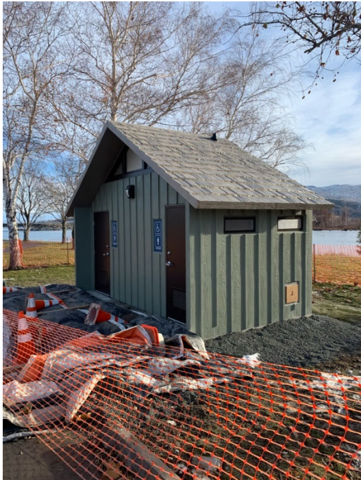
Peninsula Park Restroom
