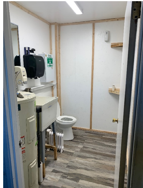
Public Works Shop Restroom
