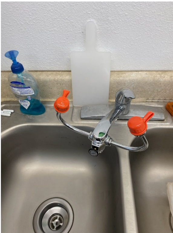
Eye wash station and GFCI outlets installed at WWTP Lab
